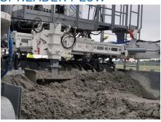
G&Z's powerful and fast concrete spreader plow is easier to change width than an auger. The spreader track sections are tapered pin connected and are light enough to be added / removed by hand with only one retainer bolt per side.
