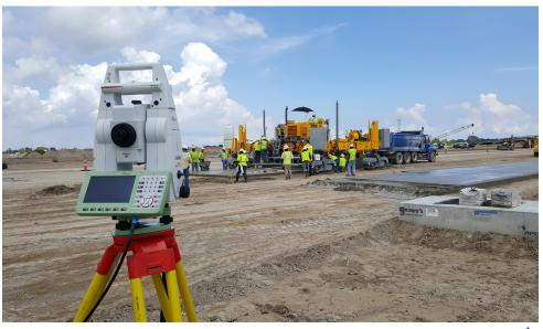
NoLine is comprised of an EGON software upgrade and a hardware mounting kit. EGON NoLine Software Upgrade integrates the use of third-party stringless technology directly into the paver's CAN Bus network.
